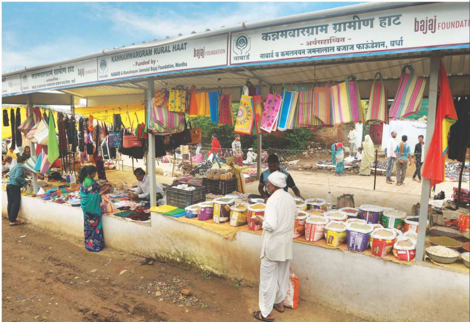
'Rural-Haat' is a dynamic platform for economic activities intending to spur economic movement; the Foundation has constructed 'Rural-Haat' at village Kannamwargram, Wardha
