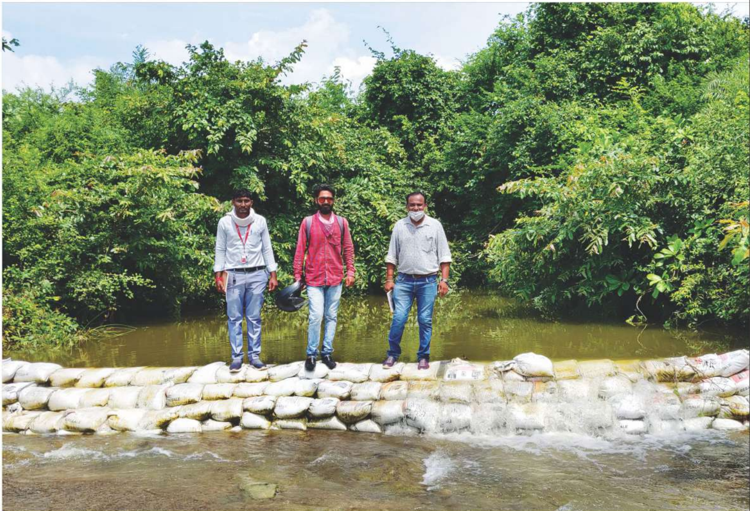
Bori-bandh is a low-cost water harvesting structure which is more beneficial to harvest the seasonal Rainwater to support irrigation to crops of rainfed farmers. 3900+ Boribahds have been established with the active participation of farmers. A boribandh constructed at village Shedgaon, Wardha
